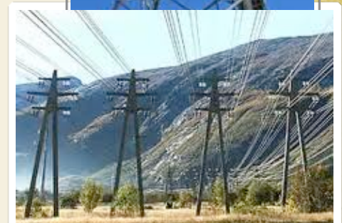
High Tension Power Lines
